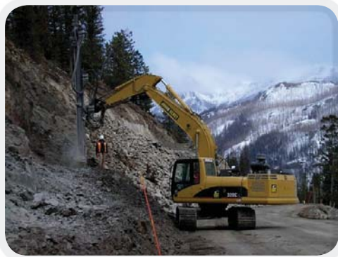
Rock Drill In Action
