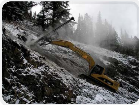
Rock Drill In Action
